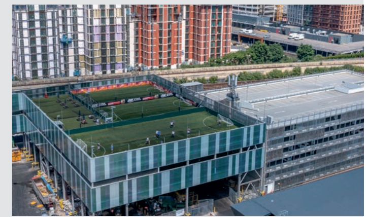
The recycling plant, multi-storey car park and Powerleague football pitches
